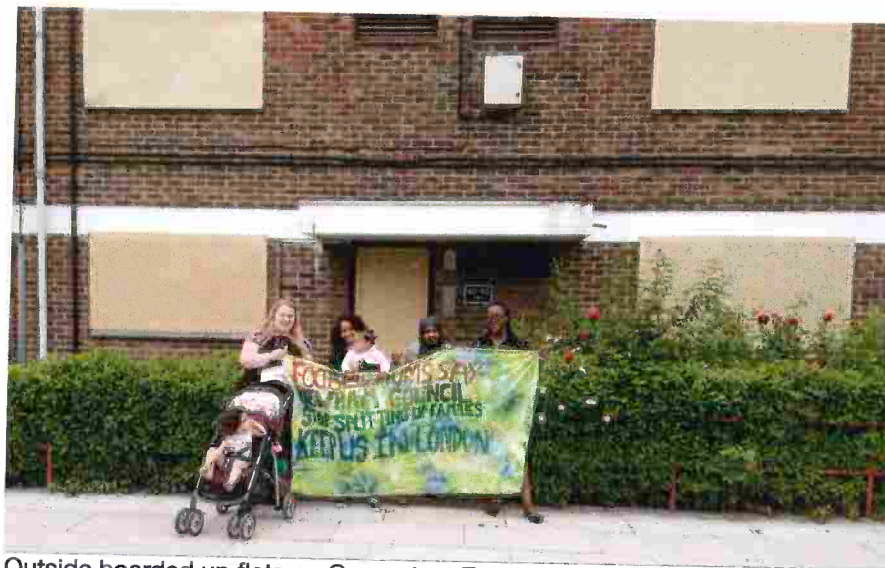
Outside boarded up flats on Carpenters Estate... Newham Council, why are these empty? They could be people's HOMES.
